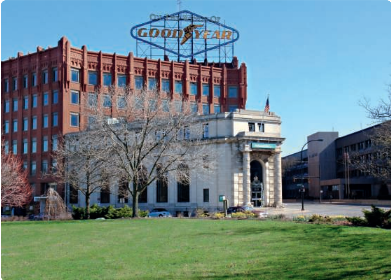
Tradition behind a well-kept brick facade: Goodyear's head office in Akron, Ohio
