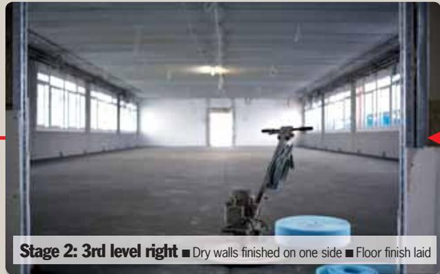
**Stage 2: 3rd level right** ■ Dry walls finished on one side ■ Floor finish laid
